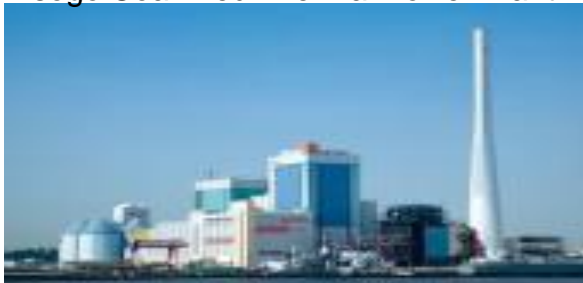
Electric Power Development: Isogo Coal-fired Thermal Power Plant
