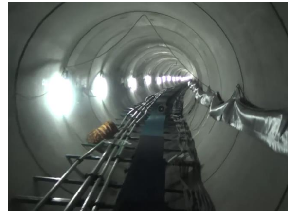
Ciliwung River discharge channel construction project
