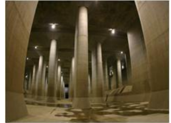
Metropolitan outer area discharge channel
